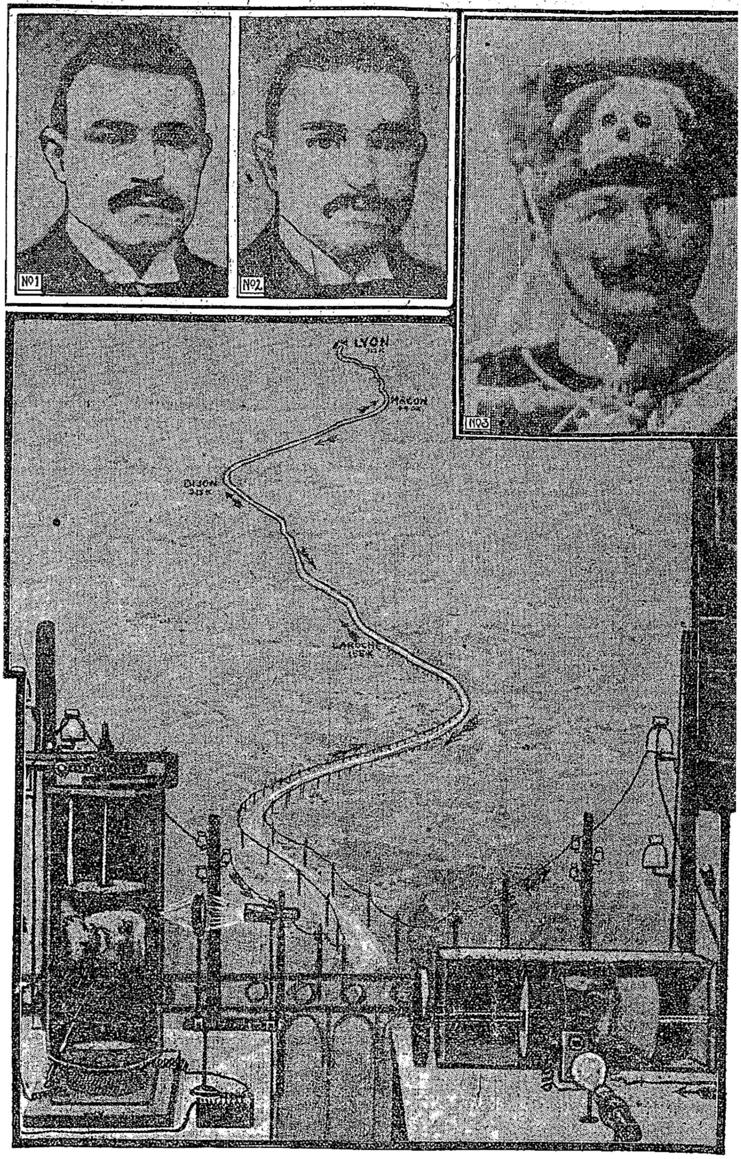
ent Fallieres Sent from the Office of l'Illustration, Paris, Over a Wire Running to Lyons and Back Again. On the Left Is the Transmitter. The Picture Is Being Received on the Right.
